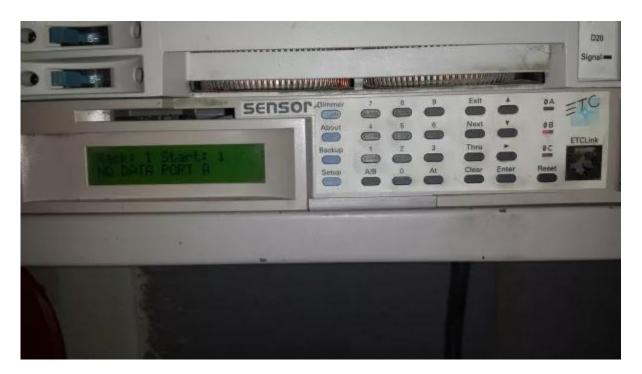
The dimmer rack and all of the lights can be controlled directly from the input section on the bottom. The LCD shows a printout of the command and status. In this photo, the rack and start mean this is rack #1 (on some big stages, you may have multiple dimmer racks), and the 2nd line indicates no lighting board
