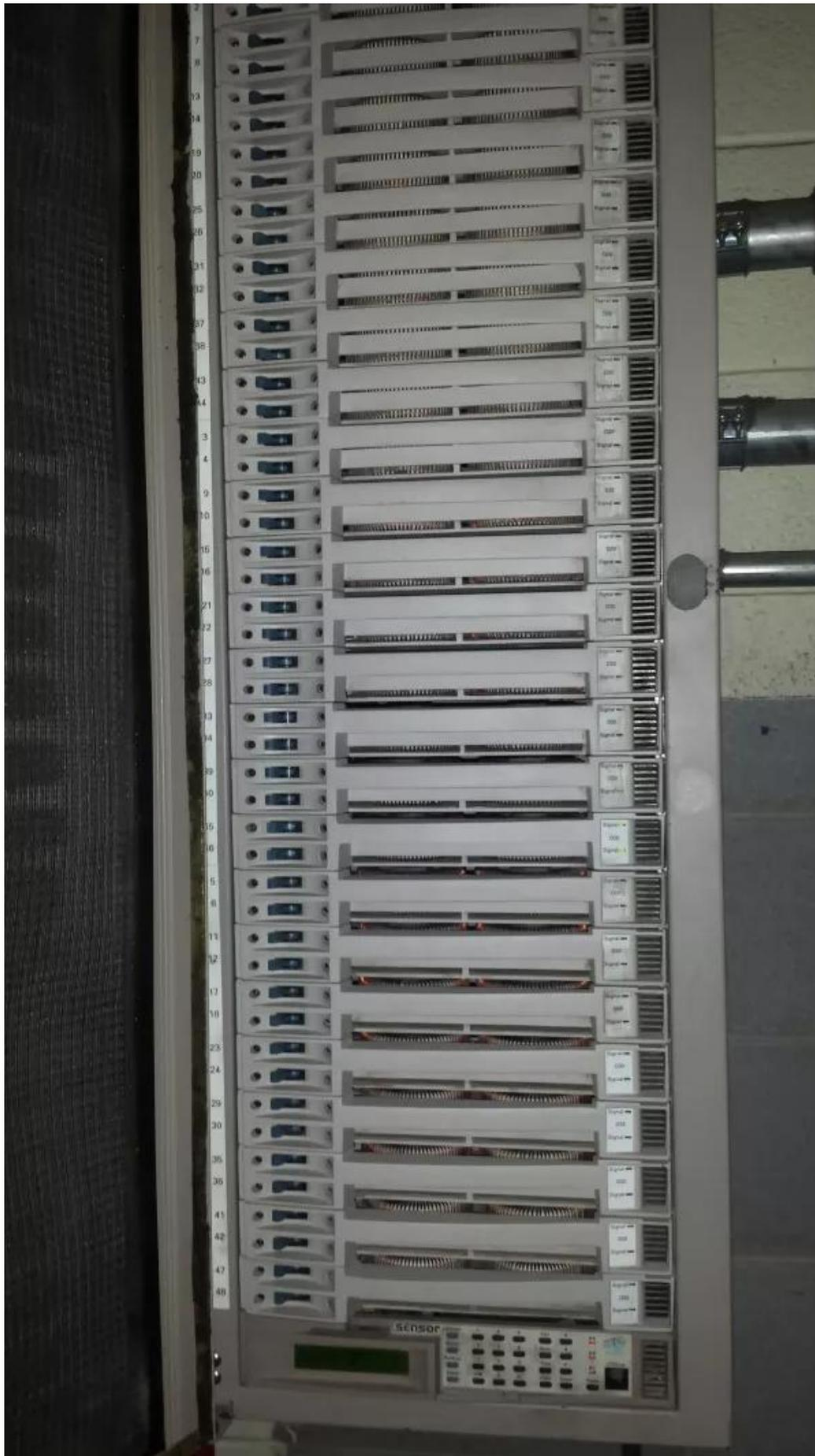
When you open the front panel, you can see the full panel. On the left side, there are the dimmer number that the slot corresponds to. These can be found on the individual slots (I'm pretty sure all the outlets for the lights are labelled, I added some missing ones). This also corresponds to the DMX channel that the port is controlled by. For example, a light plugged into plug #8 will be controlled from DMX channel 8, and is dimmed via the 4th slot.
